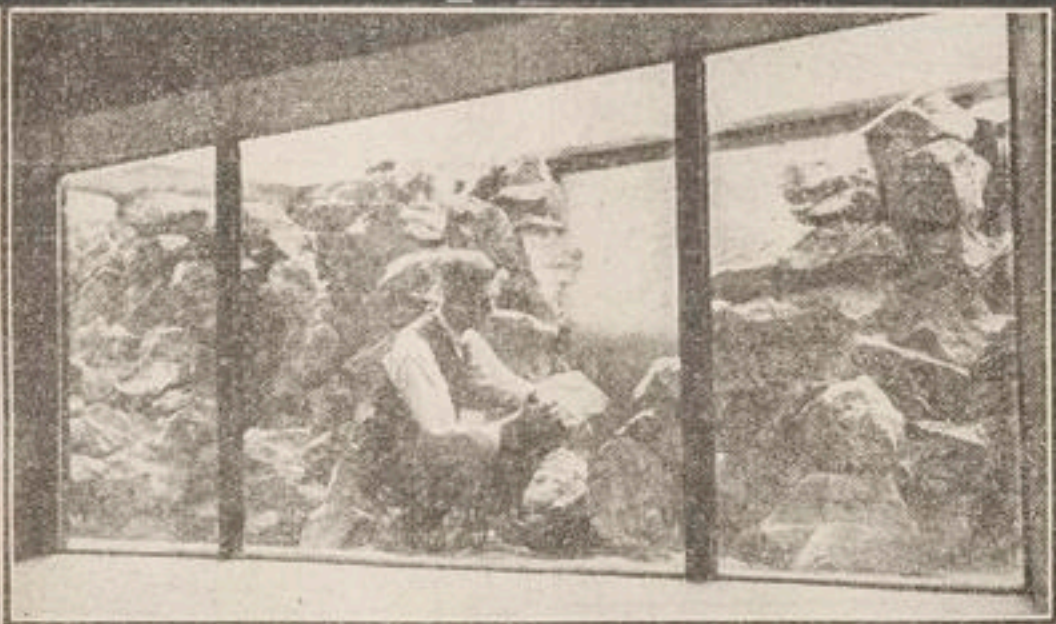
MAKING THE ZOO'S NEW AQUARIUM. — Finishing one of the two hundred tanks which are to form the new aquarium under the Mappin Terraces at the Zoo. Some of the tanks will hold thirty tons of water. — (Daily Mirror photograph.)
